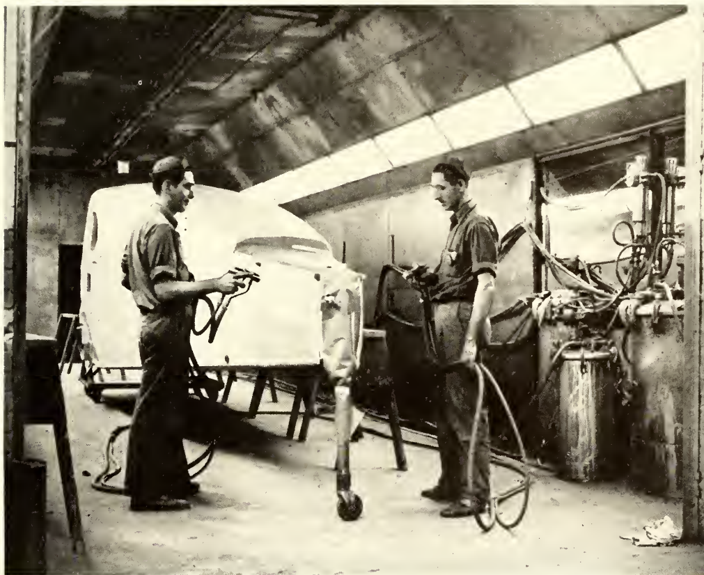
FIGURE 5-99.—Spraying a fuselage in a spray booth. Note how parts not to be sprayed are masked with paper held in place with masking tape.
